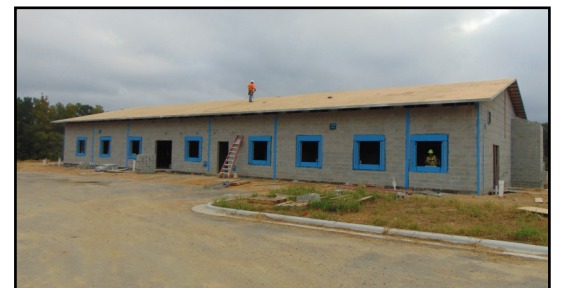
Work continued through Fall of 2019
