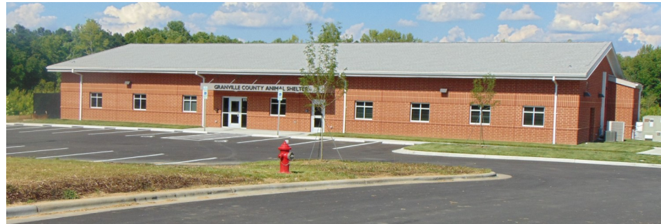
Construction completed by Bordeaux Construction, Inc.
